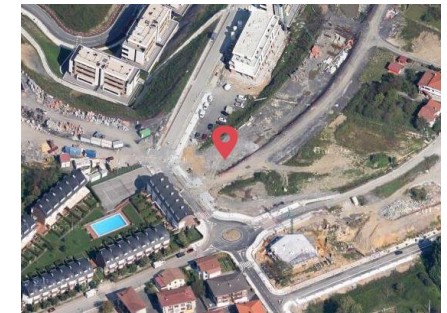
Goiegi Homes, Guipuzcoa – Construction started in Q2
